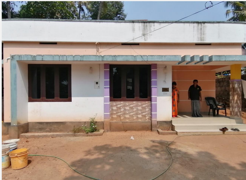
Figure 69 Completed Home of Sreemathi under CARE Scheme
