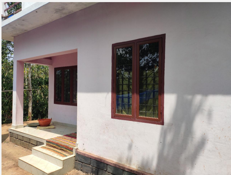
Figure 61 Rajamma's home after construction via CARE Project
