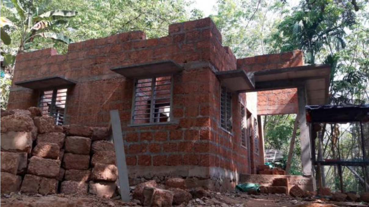
Figure 94 Images during Construction
