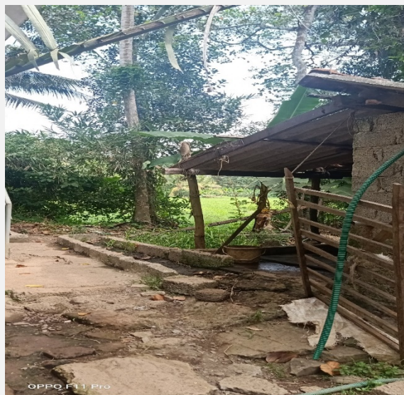
Figure 40 Collapsed home after floods
