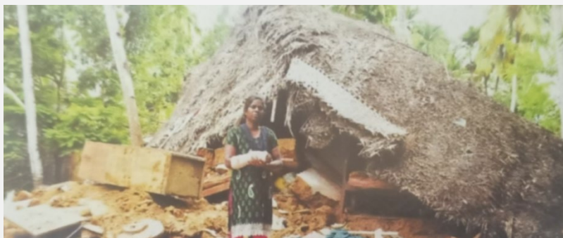
Figure 28 Radha in front of the damaged house
