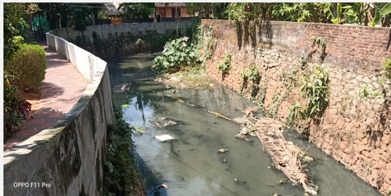
Figure 27 Amayizhanchan canal which caused flooding in the area
