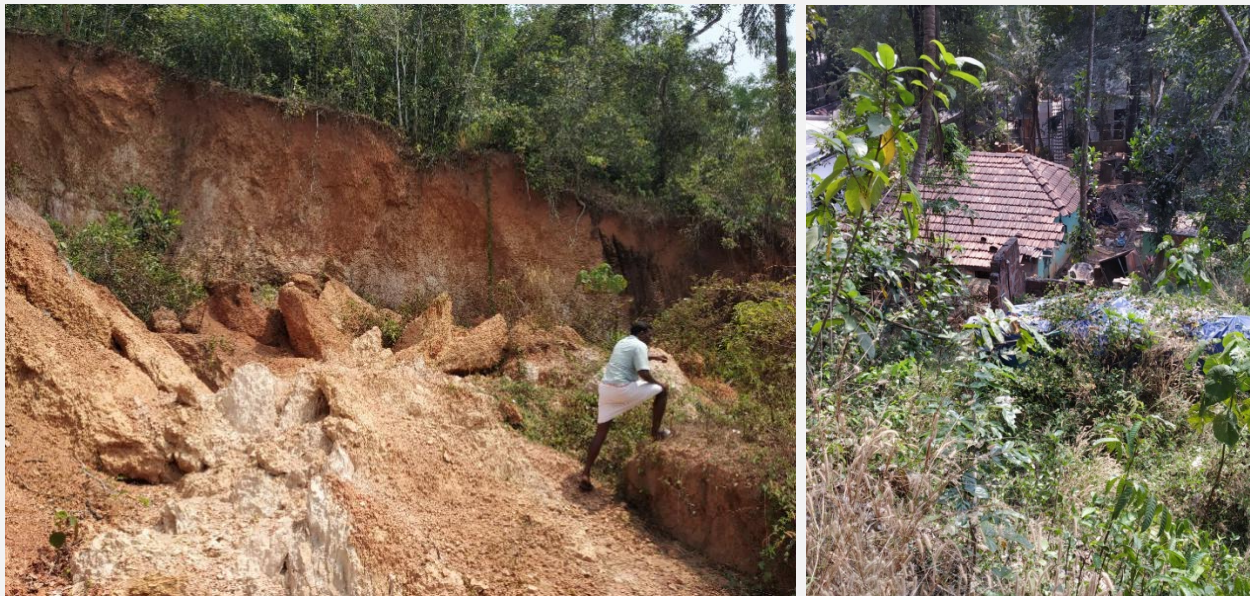
Figure 110 Remains of the damaged home and the landslides that affected that area
