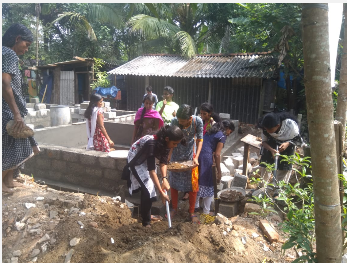
Figure 56 Voluntary support from College students while the construction of Kumari's home was ongoing
