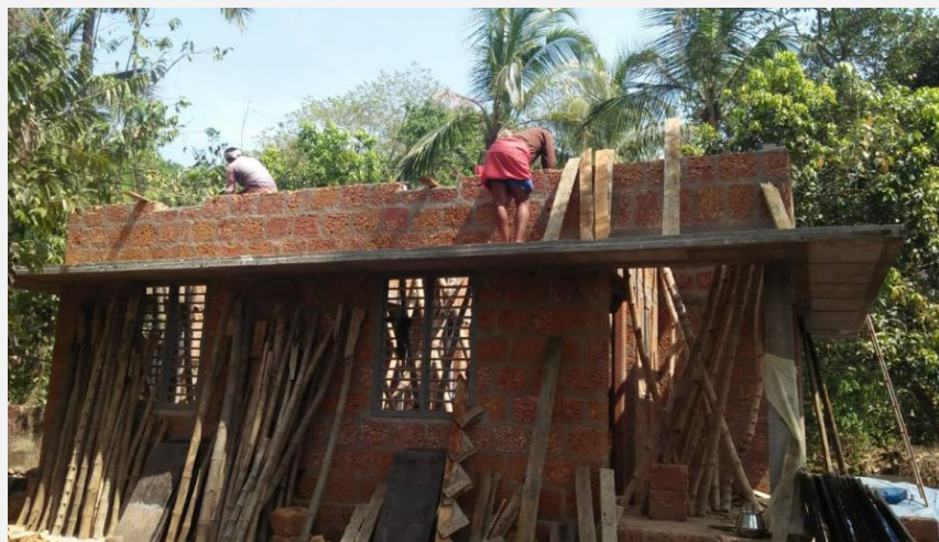
Figure 89 Image of Nabeesa's Home when construction was ongoing
