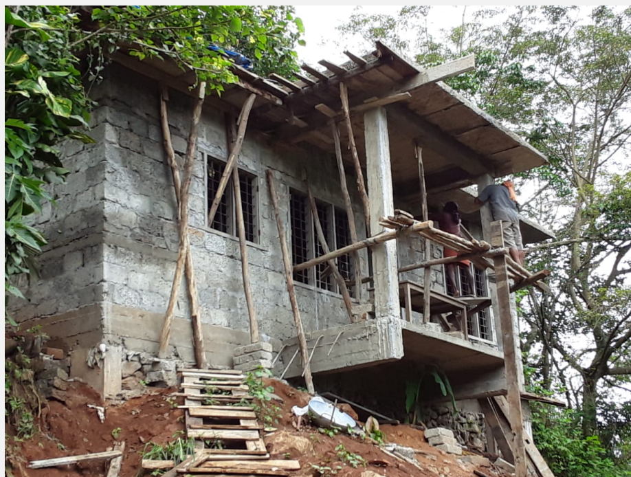
Figure 58 Babu's Care Kerala home during construction
