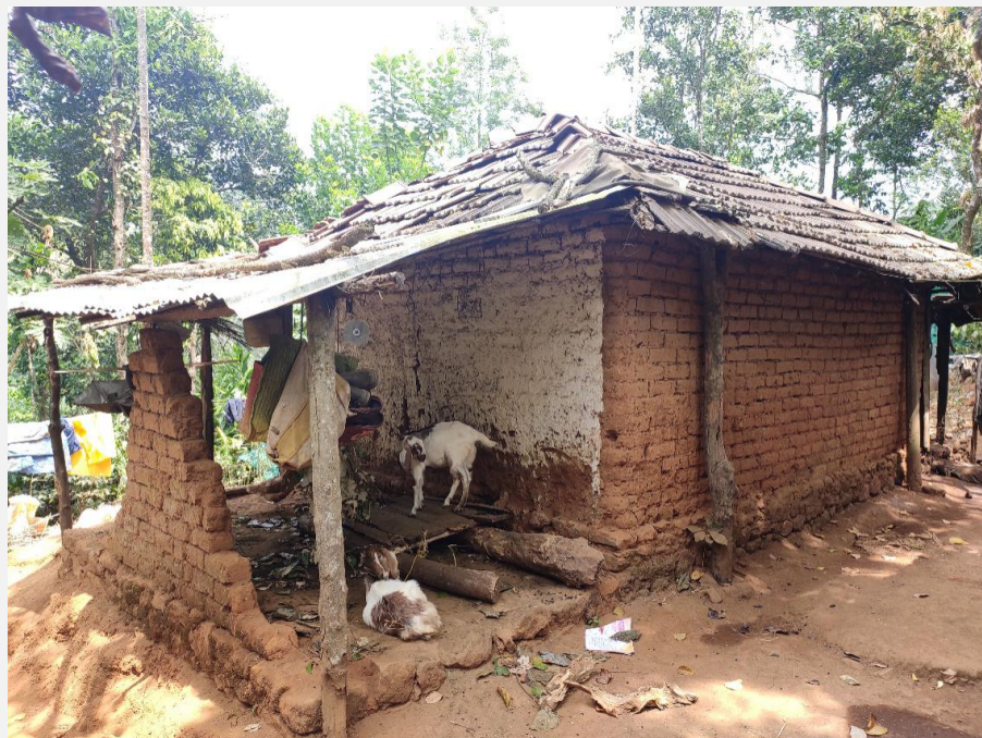
Figure 62 Rajamma's home before the floods
