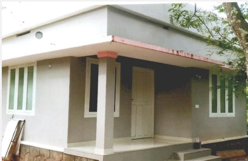
Figure 73 Newly Constructed House for Santha under CARE Scheme
