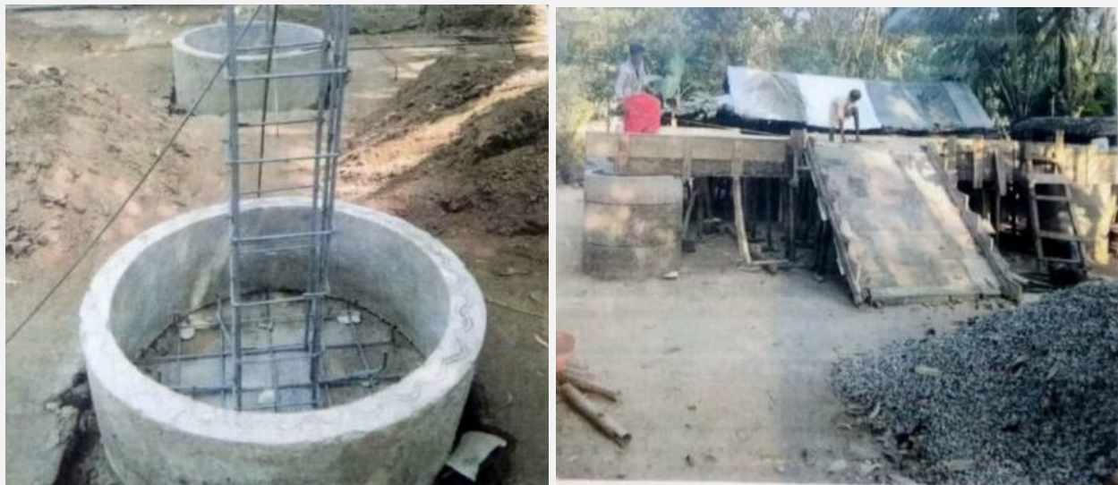
Figure 50 Different stages of Construction
